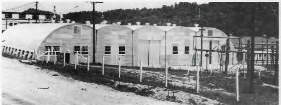
In the late 1940s the Laboratory built only temporary structures, such as these quonset huts.
