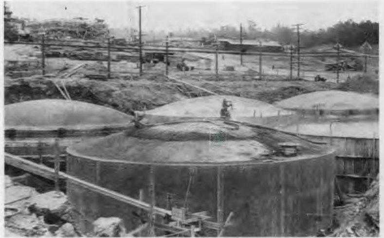
Underground tanks stored radioactive wastes from the Graphite Reactor.
