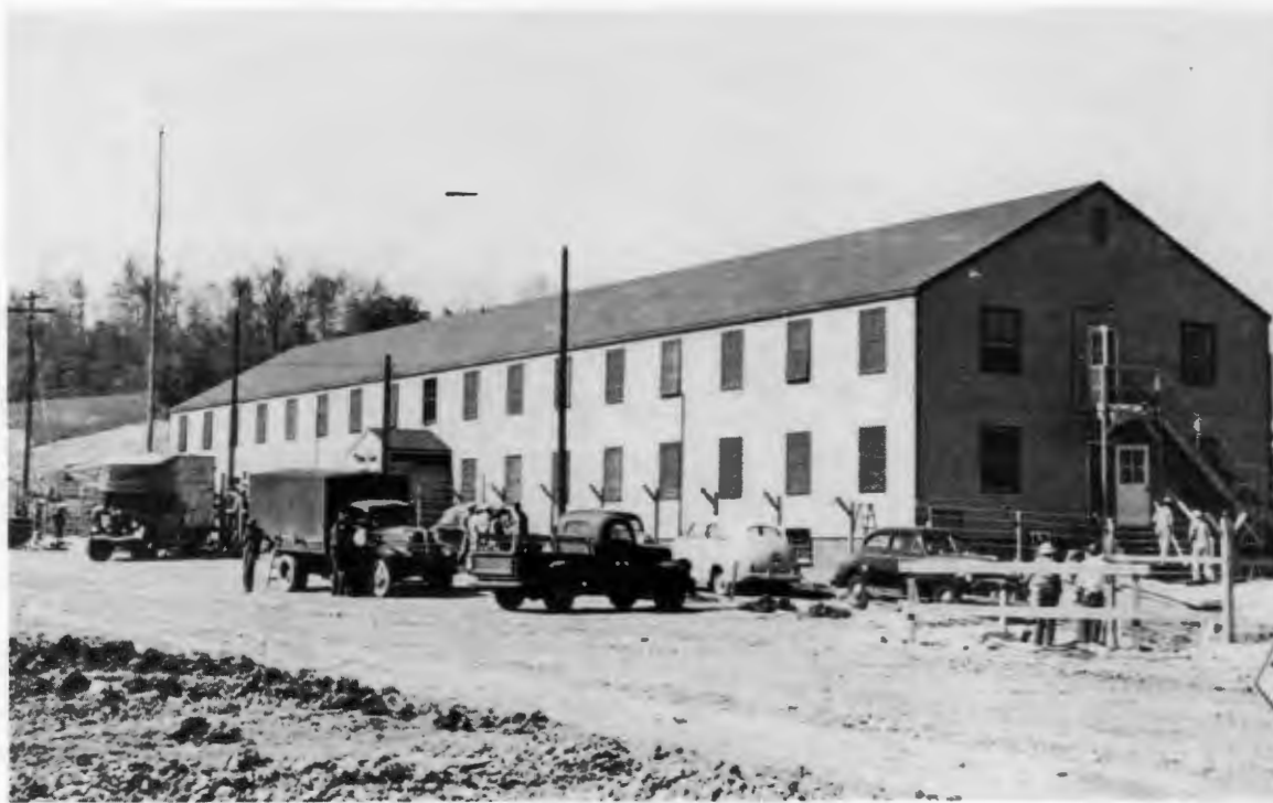
Main office building at Clinton Laboratories under construction in May 1943.
