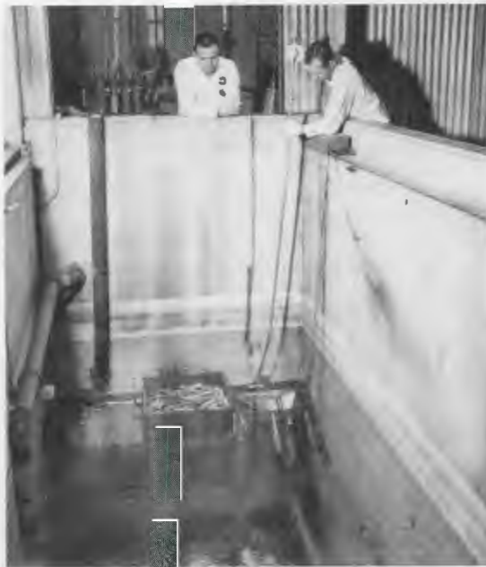
Uranium slugs encased in aluminum fell from the back of the Graphite Reactor into a canal. Shielded from radiation by the water, workers pulled buckets full of uranium slugs into the nearby separations building for the extraction of plutonium.
