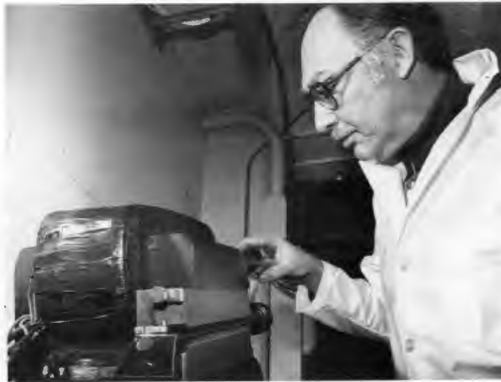
Eugene Hise pours crushed coal into a magnetic separator designed to remove contaminants from pulverized coal.
