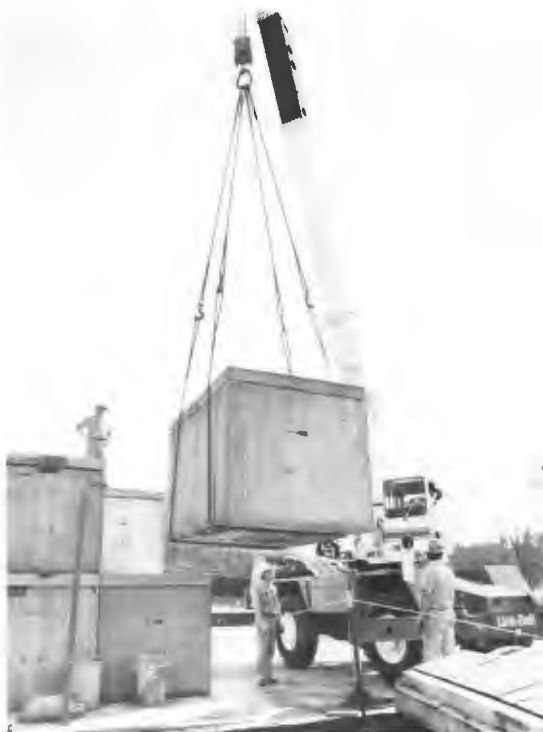
Crane hoists concrete vault containing radioactive waste into place at one of the Laboratory's engineered storage facilities.
