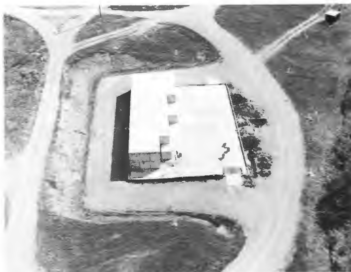
ORNL wastes are now classified and isolated in engineered storage facilities such as this "tumulus" site.
