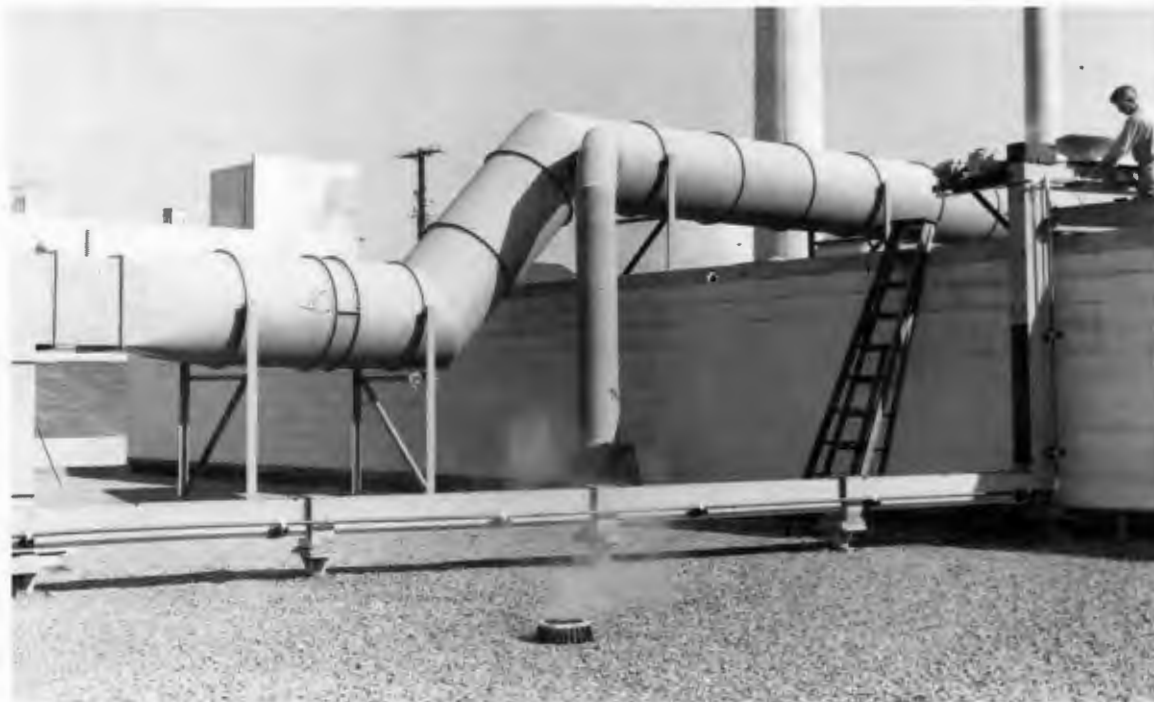
Sample conveyor on Building 3019 for the THOREX pilot plant's tests of nuclear fuel reprocessing methods.
