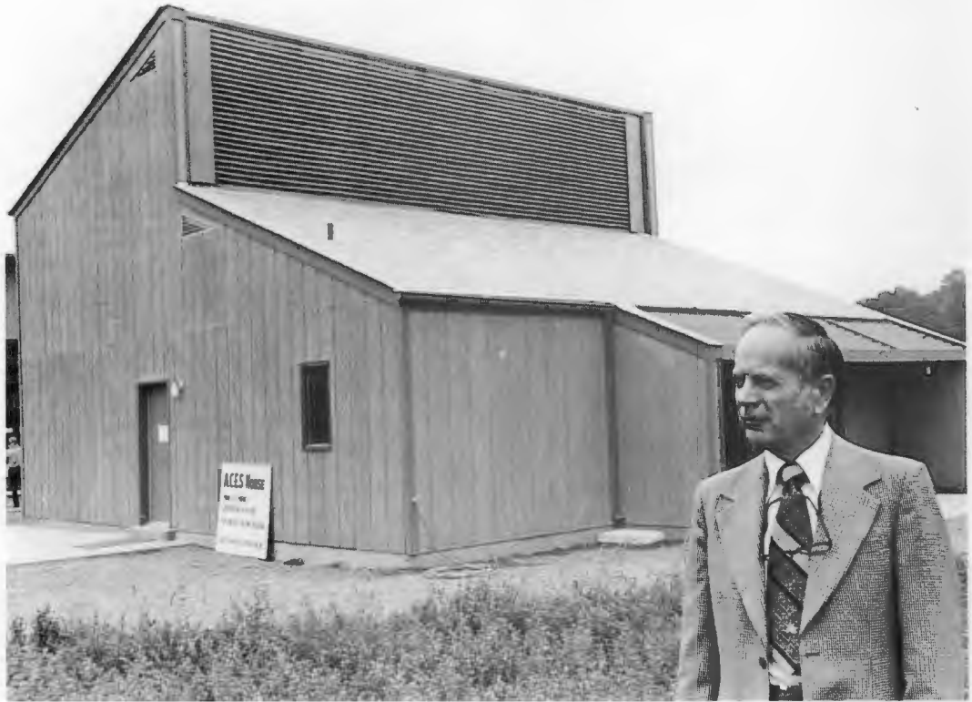
Harry Fischer stands before a house built during the 1970s to test his annual cycle energy system.
