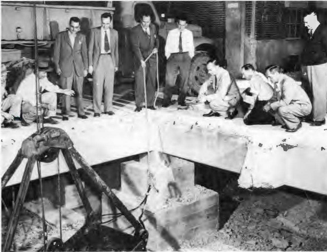
Director Clarence Larson initiates construction of the 86-inch cyclotron.
