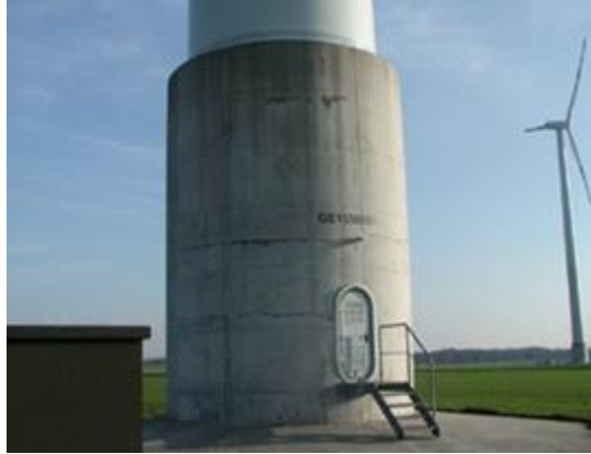
Figure 2. Concrete pedestal of a wind tower
