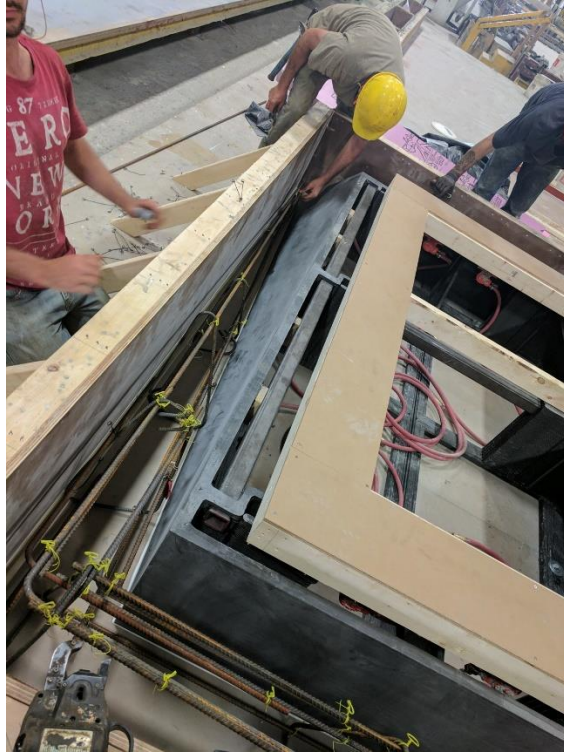
Figure 17: Installation of reinforcements
